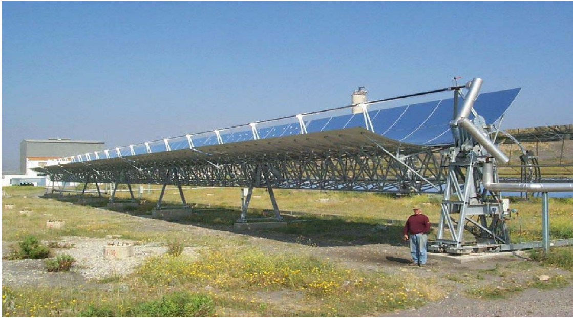
Figure 4.1: EURO-Trough collector [98]
