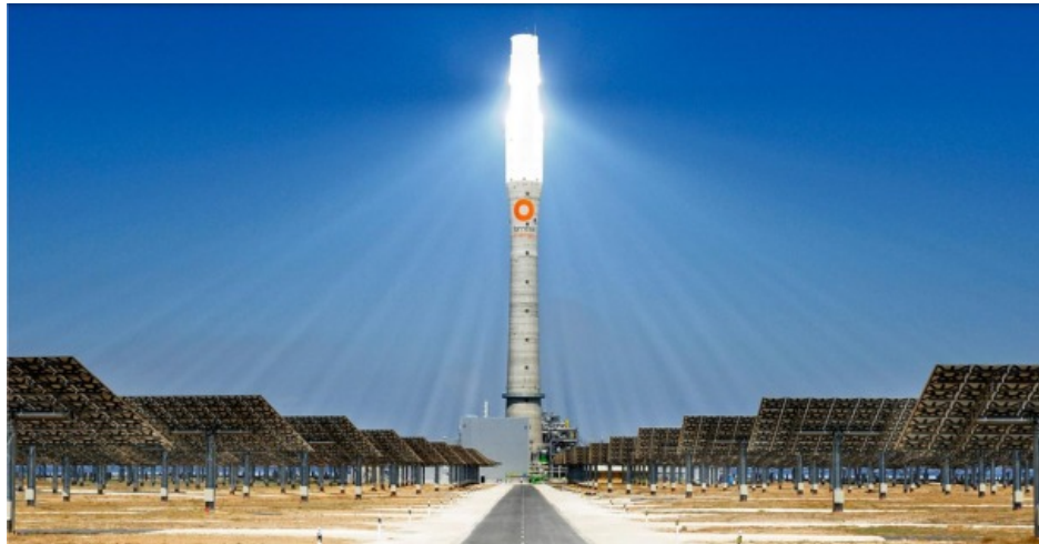
Figure 1.19: Gemasolar Concentrated solar power tower near Sevilla, Spain[58]
