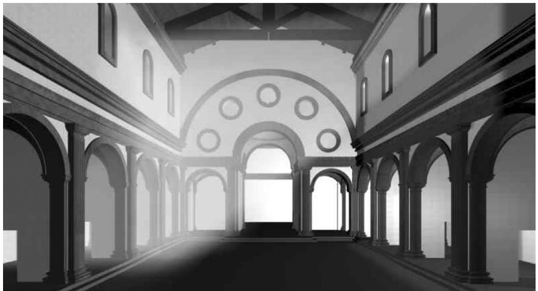
Fig. 10. Church of San Gallo. Reconstructive hypothesis of the interior, view of the chapels, coffered roofing, clerestory with single-lancet windows. Elaboration by Ylenia Ricci.
