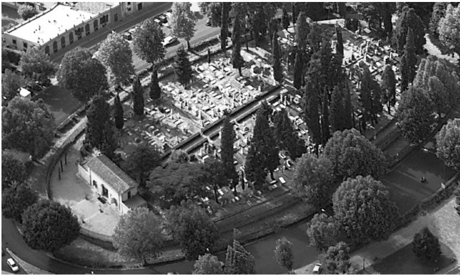
Fig.1 – Aerial photograph of Piazzale Donatello (Firenze – Italy).
