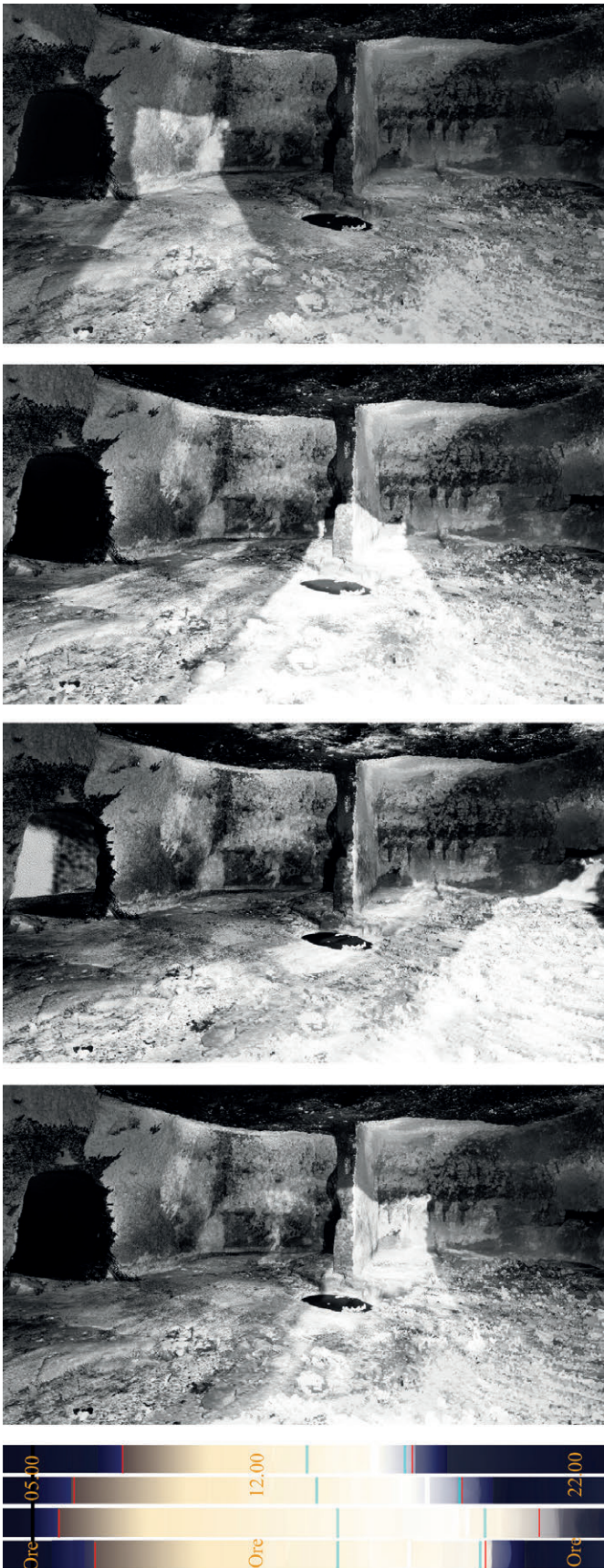
Fig. 5 – Southwest side. Cave 27, type with tuff septum. Study of sunshine. Point of maximum entry of direct light, in order, from the winter solstice to the autumn equinox. The graph summarizes the trend over the four days under review. A.A. 2022/23 (graphics E. Pieroni and F. Sini).
