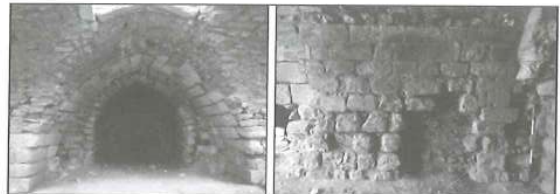
8. CF8: vaulted niche and masonry techniques (Type 3).
