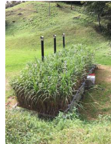
Figure 1. Photo of the pilot at Dragomer, Slovenia in September 2019. The pilot contains 9 basins in triplicates for the three of operation mode: passive aeration, draft aeration or forced aeration.
