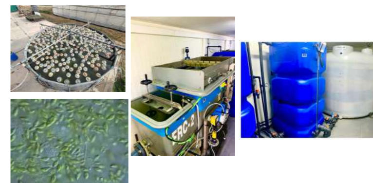
Figure 1. Photographs of the SPOT pilot plant. (A) Images of the photobioreactor (PBR) with light-pits and image (light microscopy; x100) of Tetradesmus obliquus and presence of cyanobacteria in the form of filaments. (B) Dissolved air flotation (DAF) unit. (C) Corkwood biofilter (CWF) and treated water tank.
