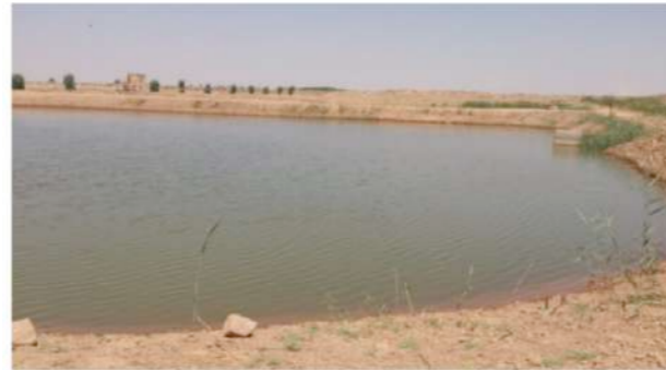
Figure 2. pool dewatered by wastewater treated by wetland method
