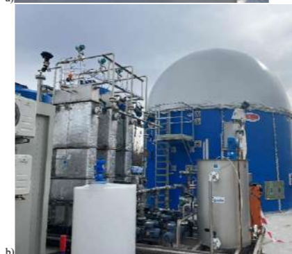
Figure 1. a) FWDs implemented in the demo plant and b) food waste dosing and AnMBR system in the Valdebebas WRRF
