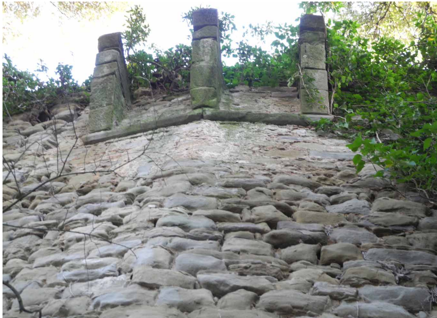
Fig. 15 Stone corbels of a sentry box in the area of the bastion between the Porta Colonia and the Porta Montanina.
