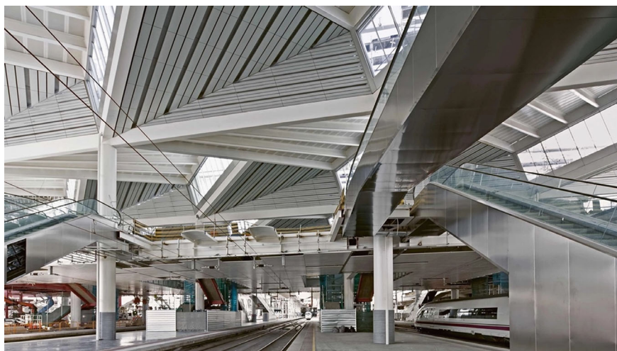
Fig. 15. new part at Madrid Puerta de Atocha train station
