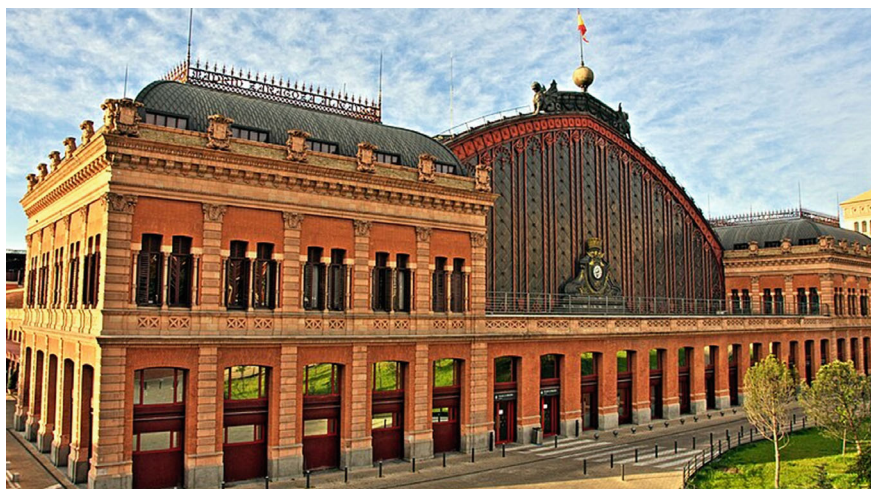
Fig. 10 Historic red brick facade
