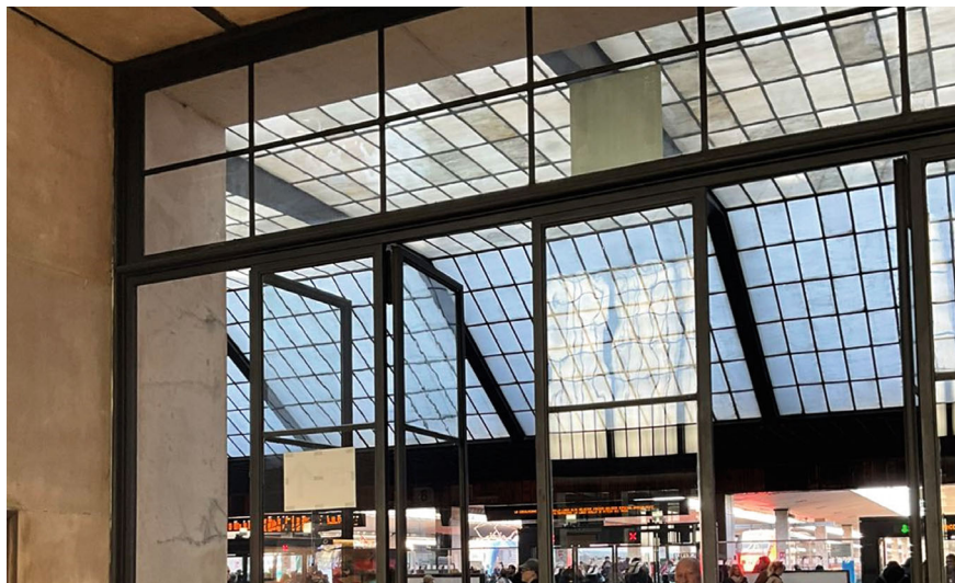
Fig. 6 Domes of modern materials such as reinforced concrete, glass and marble
