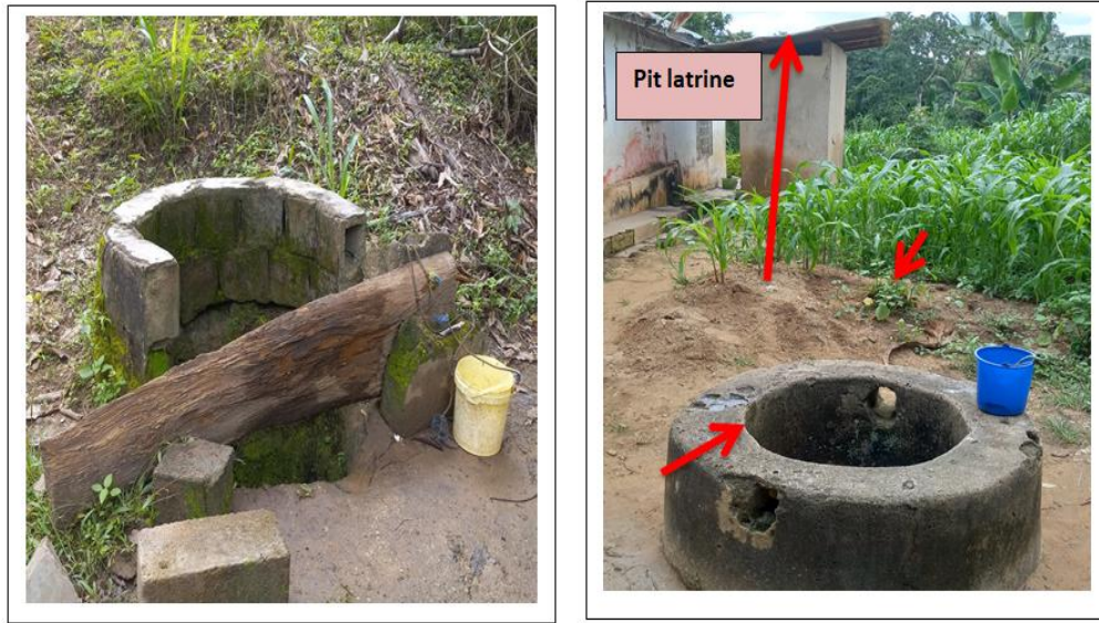
Figure IV.10b showing open, unprotected shallow wells at close proximity with pit latrines and farmlands
