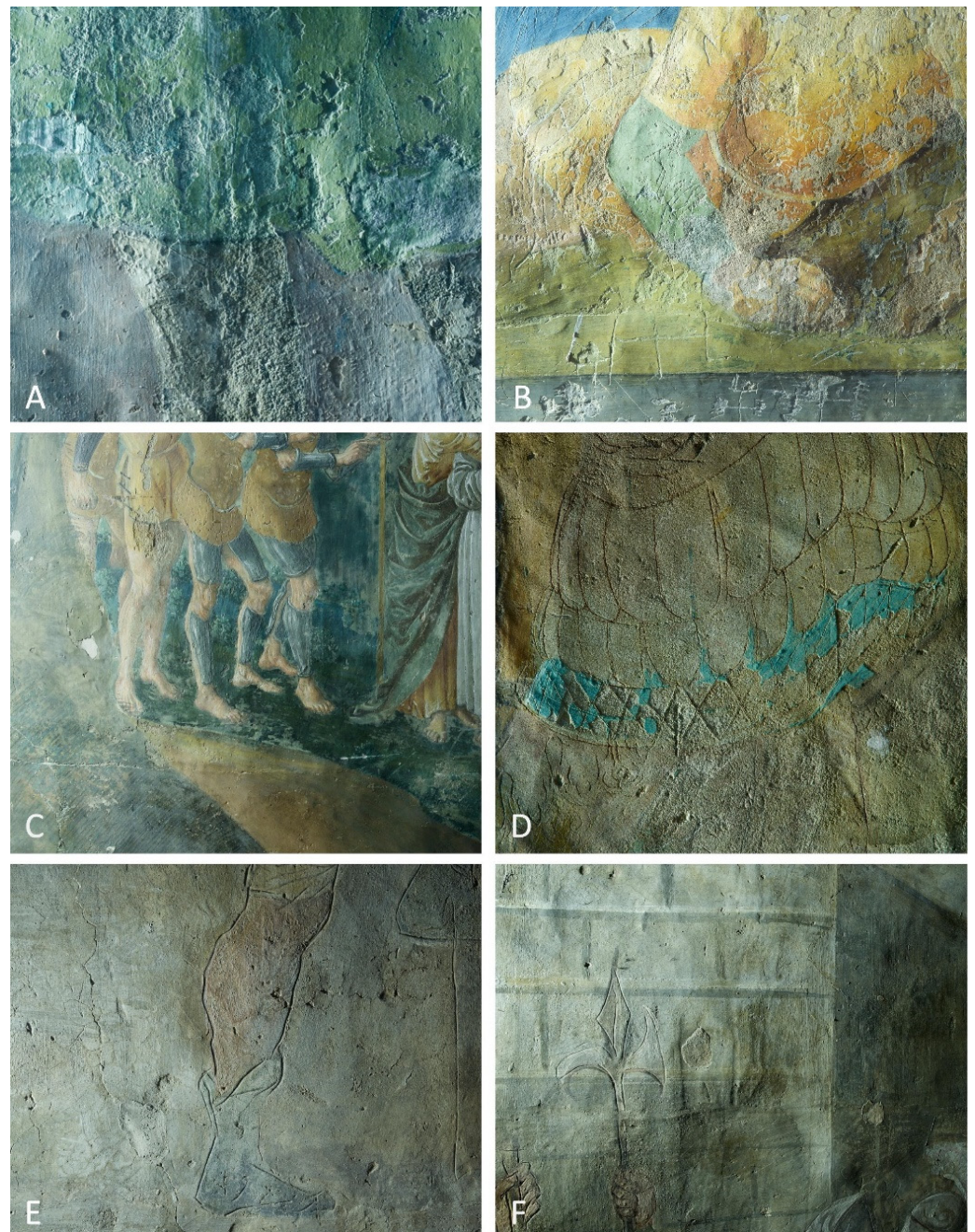
Figure 5. Raking light photos obtained on the niche (left of panel A) and panels A and B showing retouchment (A), incisions (A,D–F), loss of colours (A–D), graffiti (B), thick brushstrokes of paint and a network of small cracks (E).
