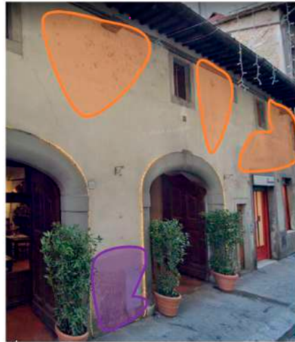
Figure 4. (From left to right)—An example of prospect and roof degradation recognition (orange area: discoloration; purple area: rising front).
