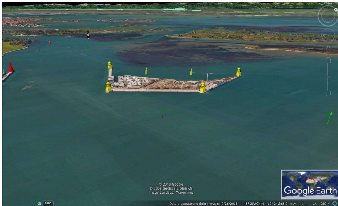
Figure 2. View of the artificial island (Port of Lido). SketchUp models simulate the expected situation.
