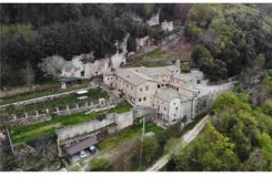
Aerial photograph of the conventual complex
