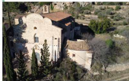
Aerial photography of the church
