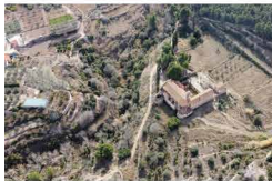
Aerial photography of the conventual complex
