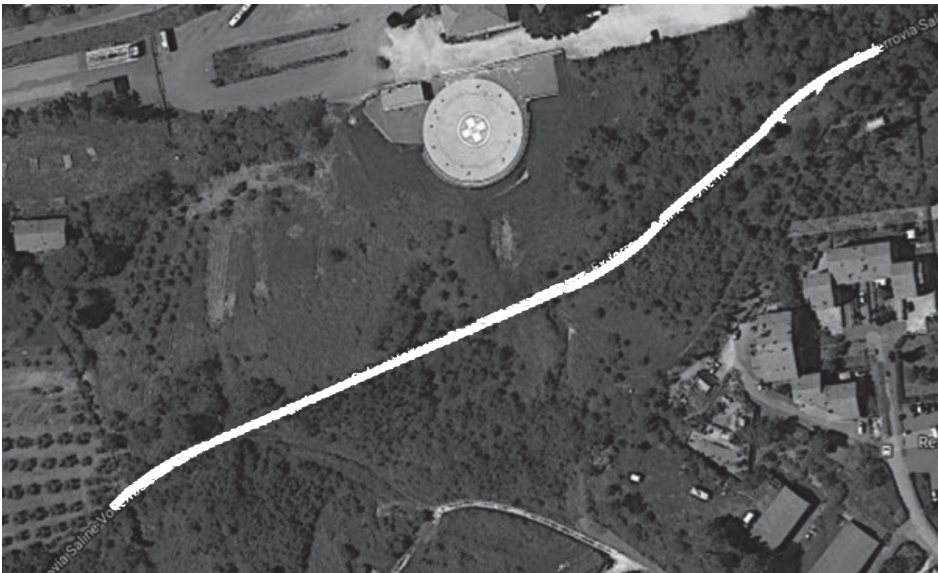
Fig. 12. Collapsed portion of line.
