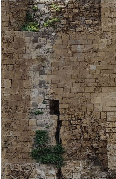
Fig. 8- A detail from the photogrammetry of the north-western front (the Authors).
