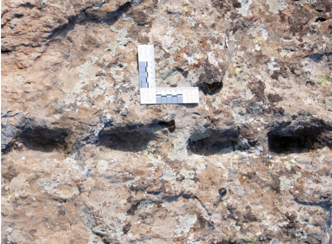
[fig. 4] Example of wedge marks
