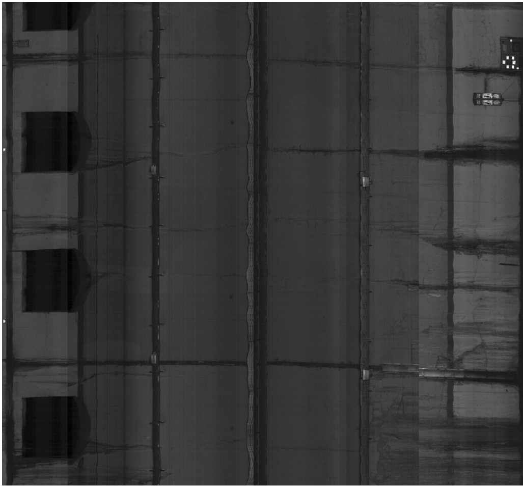
Fig. 12. Unfolded view of the tunnel block from km 1 + 180 to km 1 + 200. Minor misalignments are related to the acquisition process and do not affect the suitability of the images for inspection purposes (see Dahanayaka et al., 2026 ).
