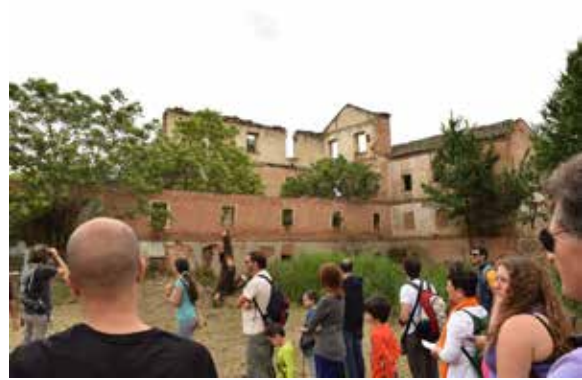
Figure 1. Community engagement to preserve UNESCO heritage and landscape in Alcalá de Henares- Spain 2018
