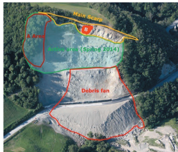
Figure 7. Aerial picture of the Vetto landslide.
