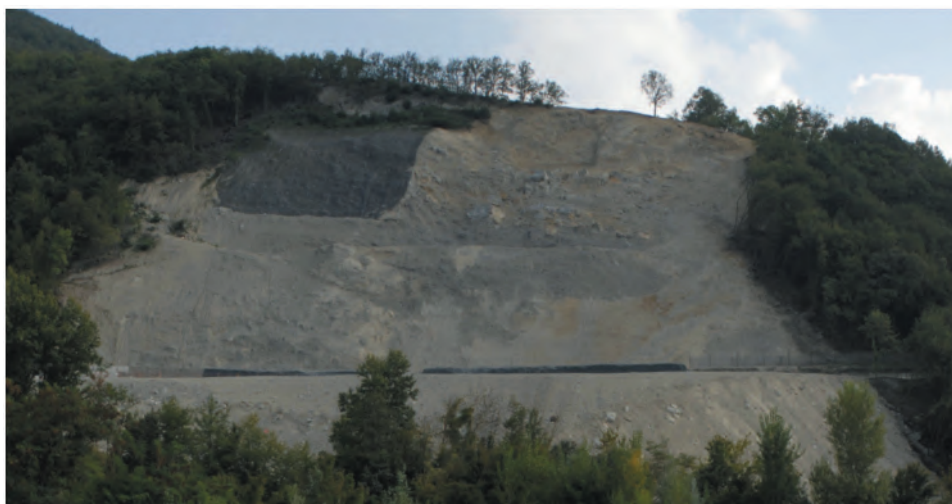
Figure 9. The landslide from the MELISSA system.
