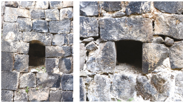
[fig. 4] Left: the single-light window on the northern side of the apse; right: the small niche on the southern side of the apse
