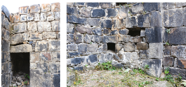
[fig. 7] Left: the new lintel replaced in the Phase 2; right: the small squared cut on the southern side
