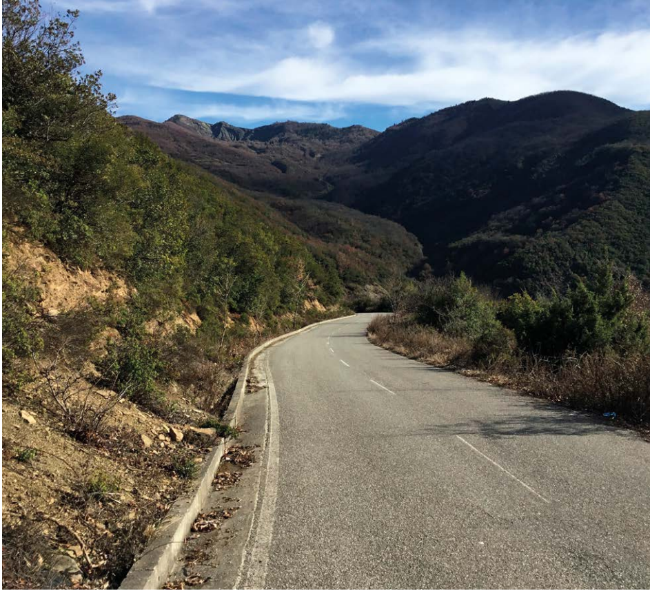
Figure 5.6 – The road up the Lëngarica on the hydrographic right of the valley to the Kadiu Bridge thermal bath area.
