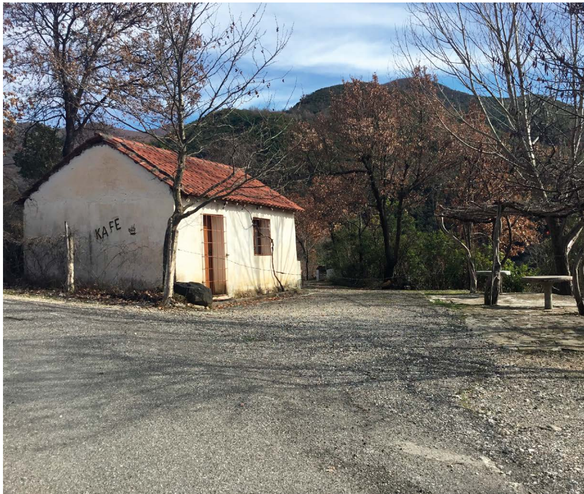
Figure 5.12 – Rest area along the valley floor road, at the intersection with one of the transversal rural routes that leads to the river only a short distance away.
