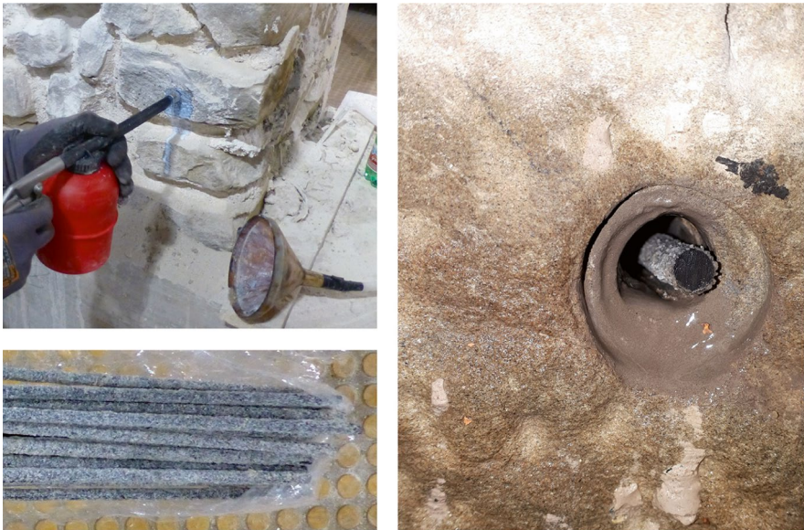
Fig. 18.11 Prototype reinforced with CC system. Reinforcement application steps
