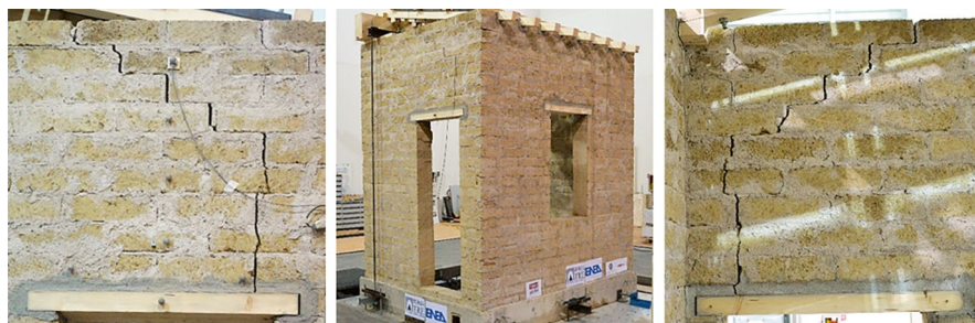
Fig. 18.4 Cracking mode of the unreinforced specimen following seismic input NRC06
