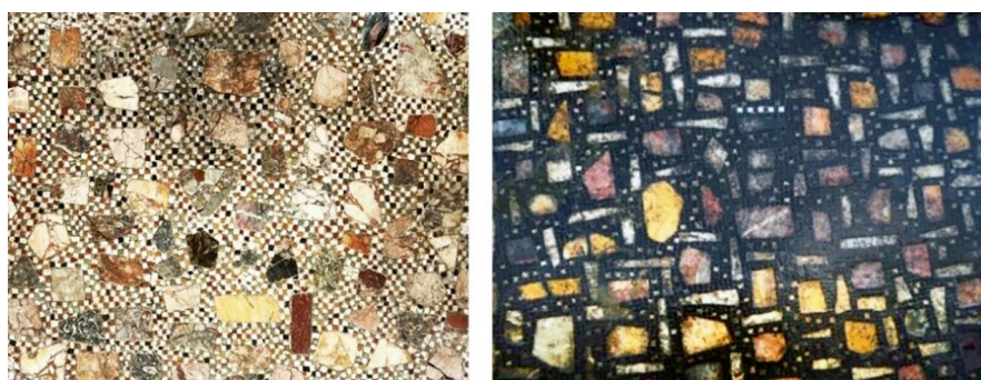
Fig. 9.3 Left: polychrome mosaic floor in the Nymphaeum—right: black dotted white mosaic floor and marble inserts in the entrance area
