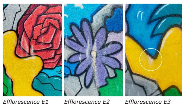
Fig. 42 Sampling areas for the efflorescences E1, E2, and E3.
