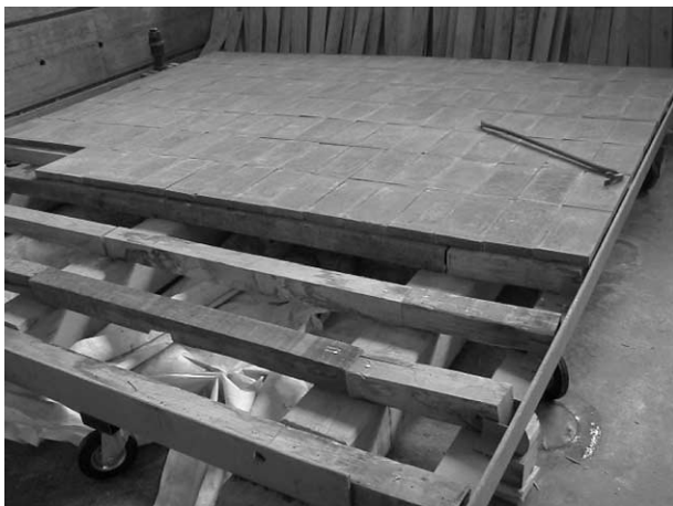
Figs. 2 and 3. Wooden beam floor with solid bricks.
