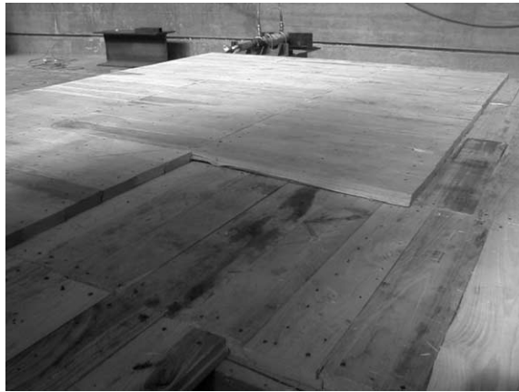
Figs. 4 and 5. A traditional reinforcement: application of an additional layer of planks.
