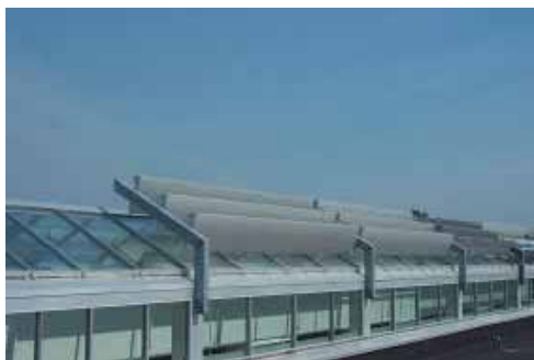
Figure 5 Shading devices at Aabenraa Hospital.
