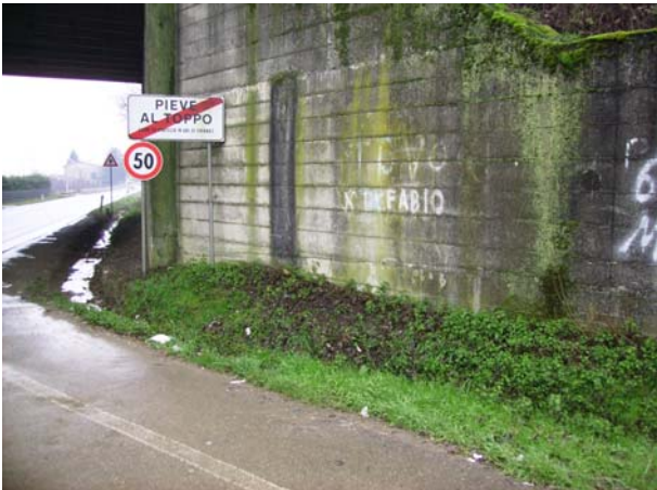
Type G – Overpass
