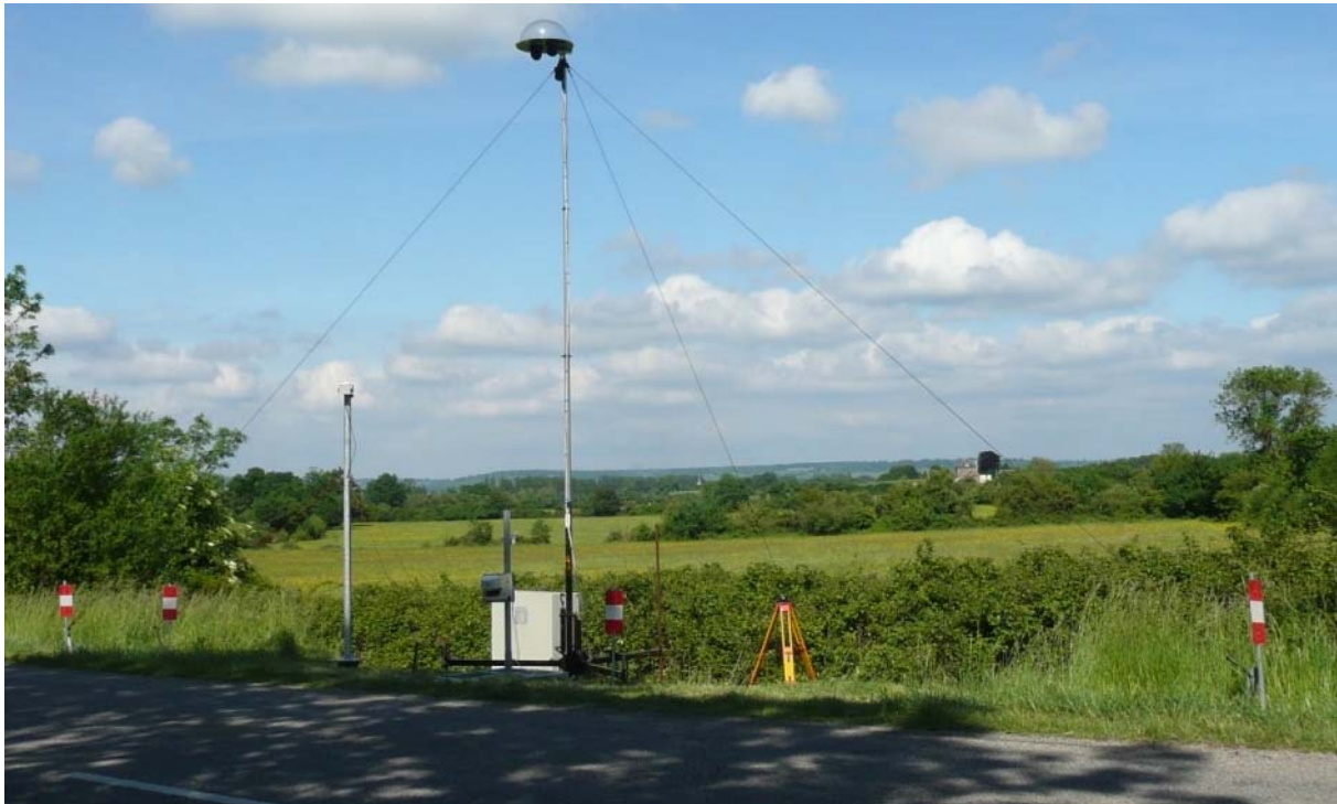
Figure 4. Installation of the OT tool
