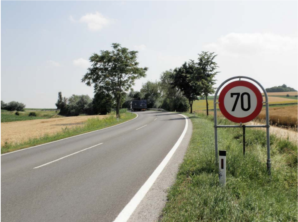
Figure 3: Accident high-risk site A [Own Picture]
