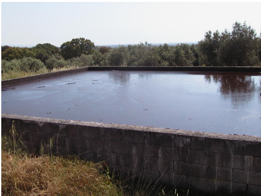
Fig. 3. Collecting pool for olive oil mill wastewater in a Tuscan mill.
