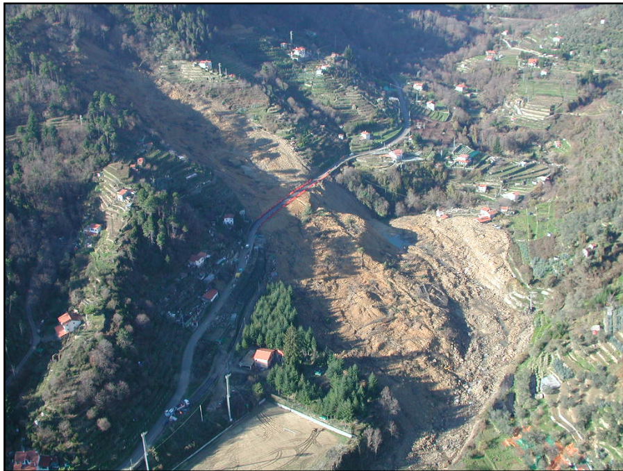
Figure 1.9: The Bestagno landslide which damaged the provincial road n°55 and killed two people.
