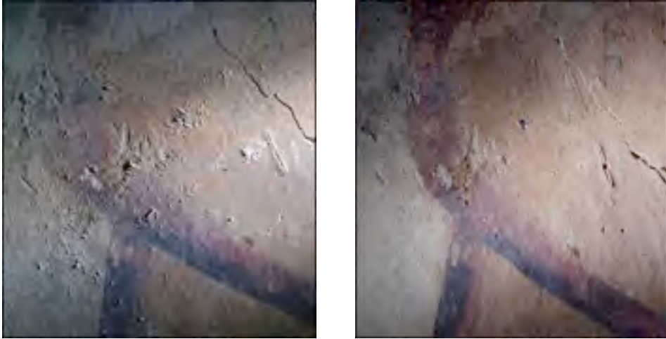
Figure 4. A detail of a fresco situated in Calakmul. On the left, before the restoration, the salt efflorescence damaged the wall-painting. On the right, the restored image.
