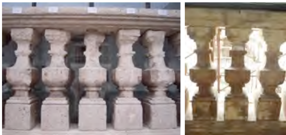
Figure 4.21. The treatment with nanoparticles of calcium and magnesium hydroxide simplified the plastering of balaustrini of Angera stone.
