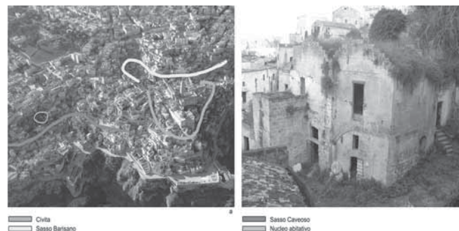
Fig. 1. Location of the residential complex within the Sassi of Matera
