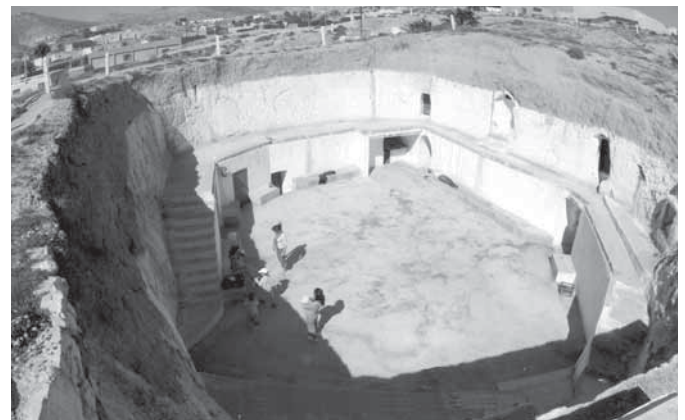
Fig. 12. Nouvelle Matmata and well house, near Nouvelle Matmata
