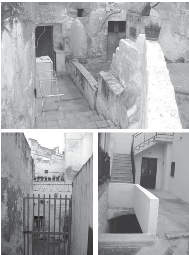
Fig. 11. well houses' transformation, Massafra (TA), Puglia
