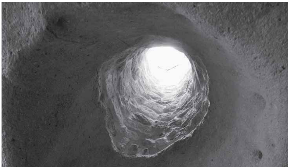
Fig. 2 Veli Toren house, Urgup: ventilation duct
