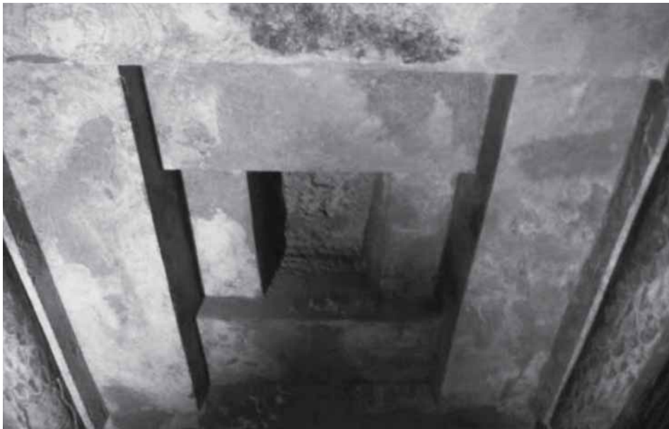
Fig. 1 Dome excavated in the rock, simulating timber corbelled construction, in the Tomba Francois at Vulci
