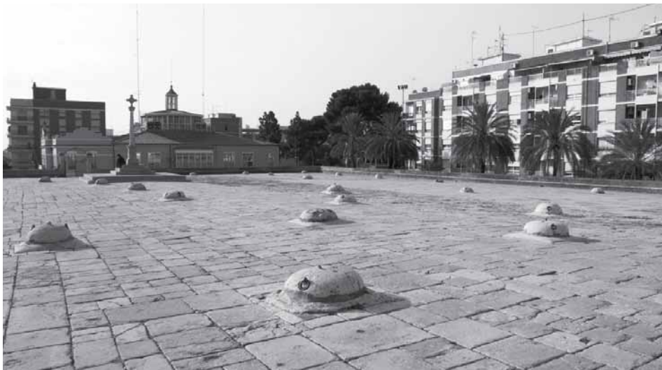
Fig. 1 The paved terrace that crowns the upper part of the silos (H. Costa)
