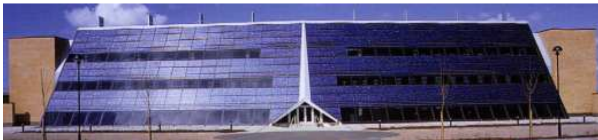
Solar Office, Doxford, Irghiltenra
