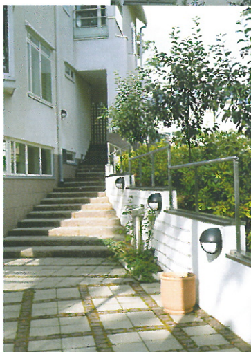
Luxury apartment building in Helsinki equipped with an underfloor heating / cooling system (free cooling energy is taken from the ground)
