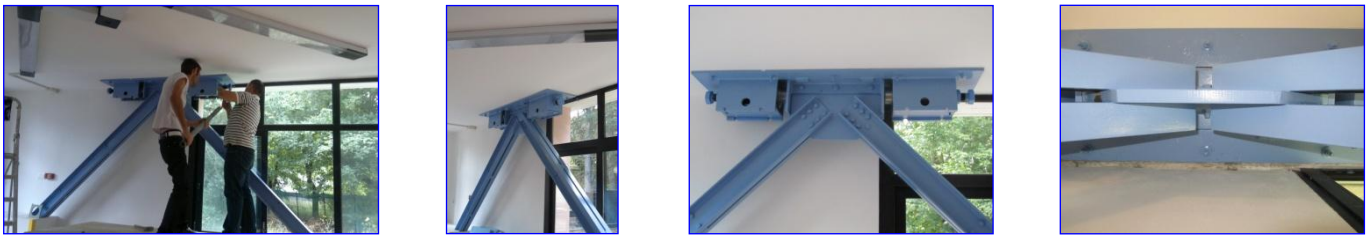
Fig. 21. Final half-stroke positioning of a spring-damper, and views of the same DB panel.
