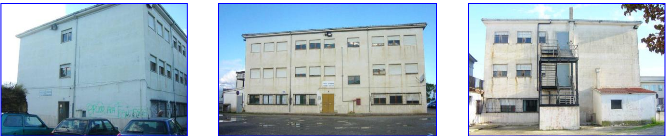
Fig. 1. Views of the building.
