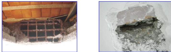
Fig. 3. Cross-section of the under-roof floor obtained by local demolition, and scrapes highlighting the bars at the intrados of a joist.
