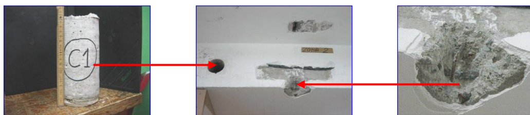
Fig. 2. A carrot extracted from a primary beam, and scrapes highlighting the reinforcing bars of the same beam.
