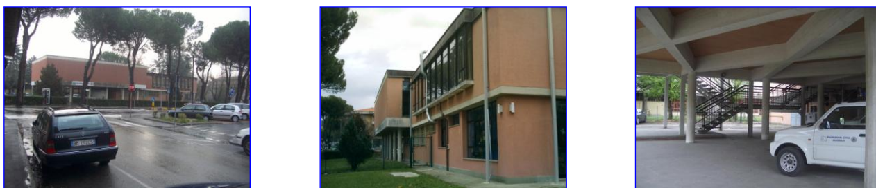
Fig. 12. Views of the building before the seismic retrofit and architectural renovation interventions.
