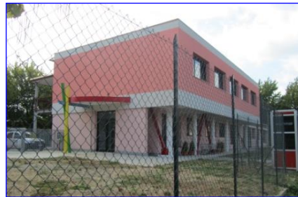
Fig. 22. View of the building after the completion of the retrofit and architectural renovation works.
