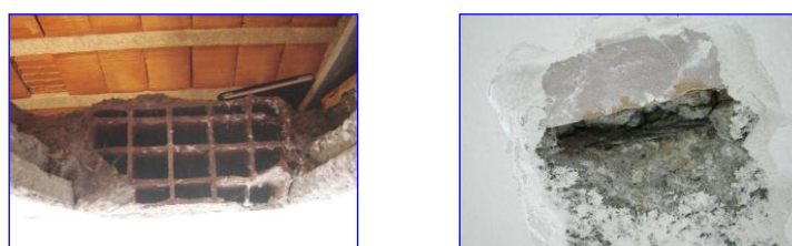
Fig. 3. Cross-section of the under-roof floor obtained by local demolition, and scrapes highlighting the bars at the intrados of a joist.
