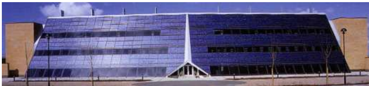
Solar Office, Doxford, Irghilterra
