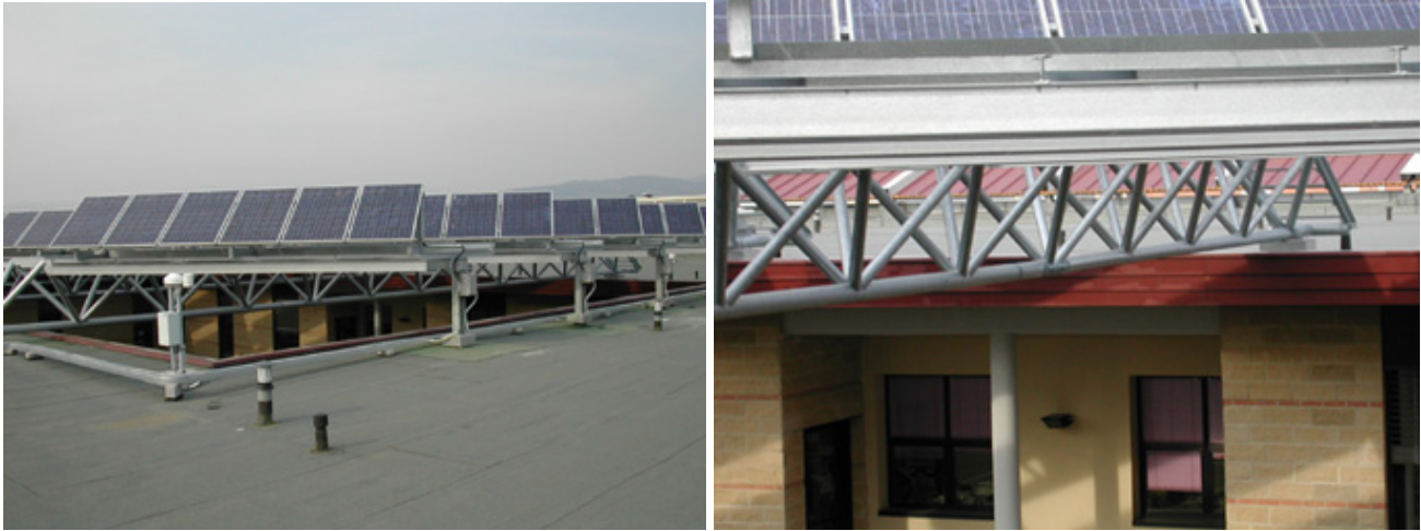
Figure 6. (a,) View from the roof (b) Detail of the structure
