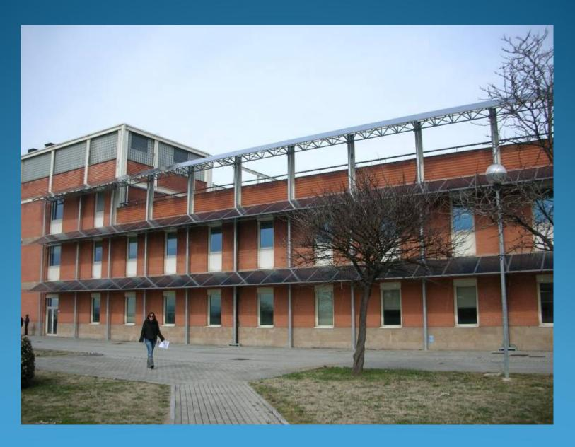
The Pv integrated system is a 50 kWp divided in two systems, one in the façade and the second in the roof as shading devices.
