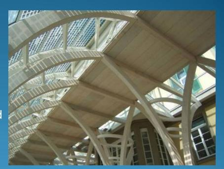
PV-laminates (size 220 x 100 cm) are arranged in parallel rows, supported by the main structure and along the vertical axis. Horizontally connected by means of the crosspieces of the structure, however, placed in the intrados of the greenhouse, ensure a continuity of composition and structural of the glass surface in the outer part.
