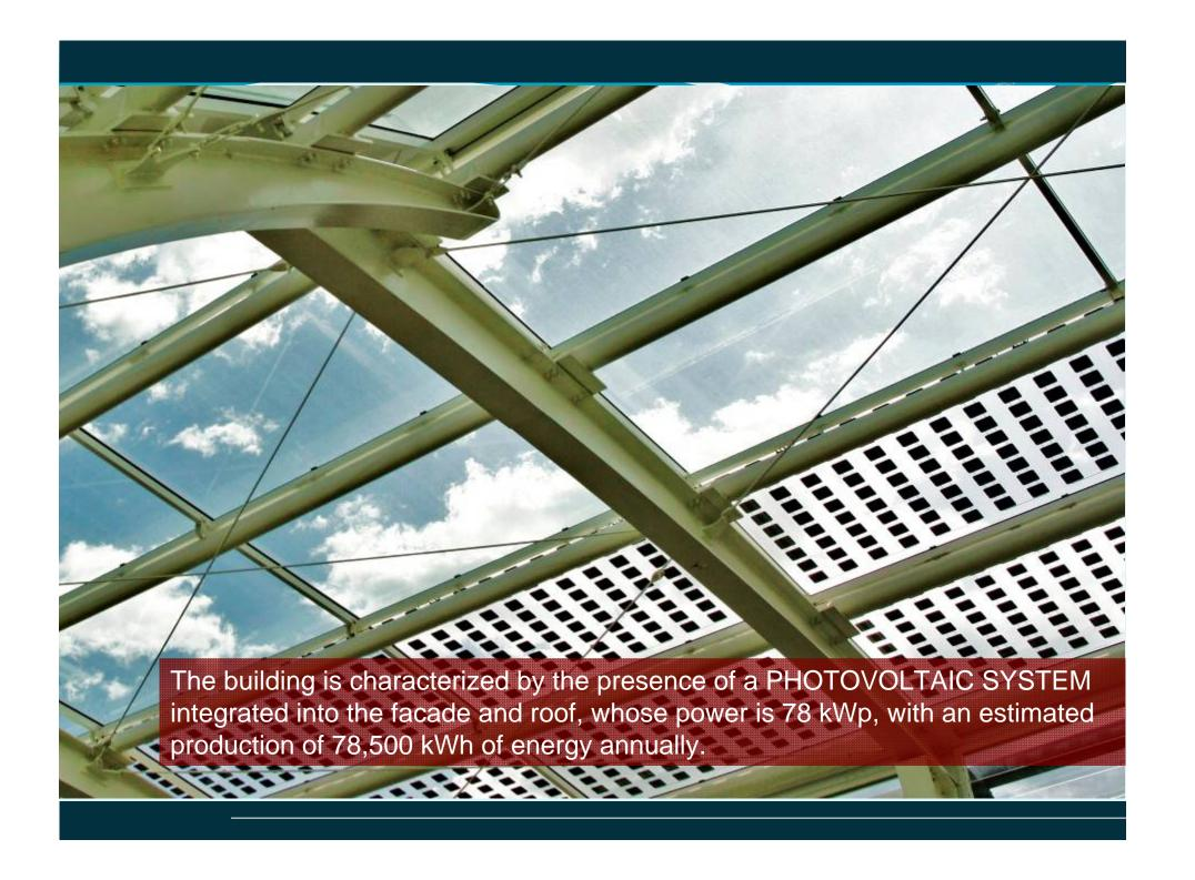
Photovoltaic cover glass (greenhouse).
