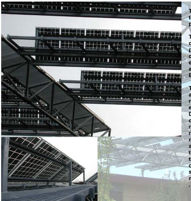
The photovoltaic modules are tilted at 35 ° in the horizontal plane and facing south.
