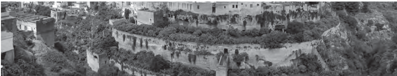
(Pic. 11) San Marco ravine: view of ponte nuovo, (C. Crescenzi).
