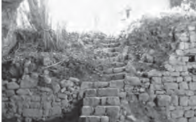
(Pic. 109) Ripafratta: Hermitage of Rupecava, (web photo).
