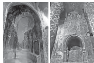
(Pic. 22 - 23) Eski Gümüşler. Church apse and left wall, (C. Crescenzi).
