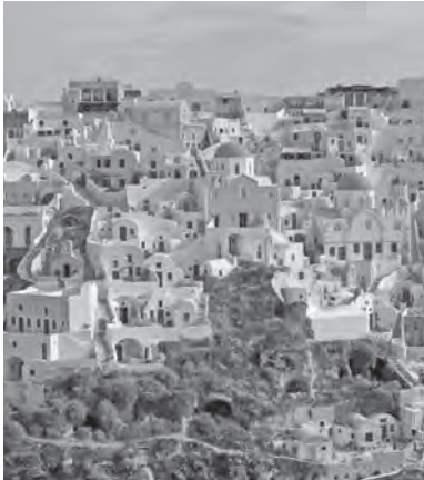
(Pic.4) Rupestrian houses "Iposcafi" and new constructions (C. Crescenzi).
