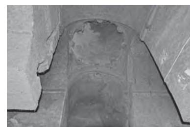
(Pic. 88) Saklı Kilise central dome of the cross inscribed church, (C. Crescenzi).
