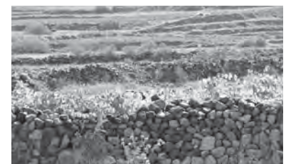
(Pic.5) Drywall able to retain rainwater and protect crops from strong winds, (C. Crescenzi).
