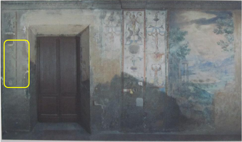
Fig.4.30: Casina Farnese: the lower loggia's fresco “ The story of Hercules and Cacus ”, before treatment. The yellow box indicates the area chosen for the trial.
