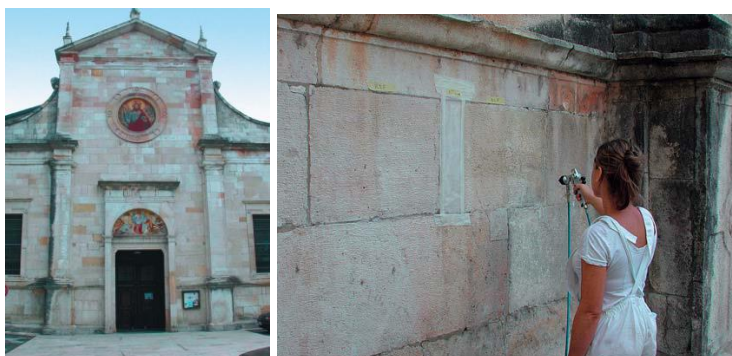
Fig. 1.3: – Church of Santa Maria in Angera: Facade of the church (left) and application of the spray solution of BCF (right).
