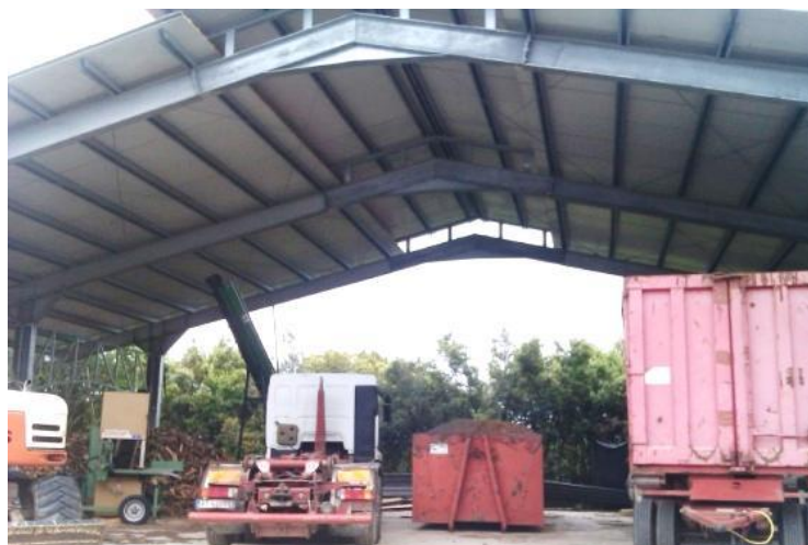
Figure A-6: Area equipped with biomass pre-treatment machinery
