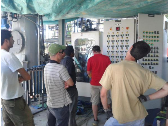
Figure 6-6: Research team and technician at control panel for last check before system start-up.
