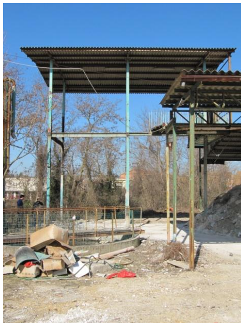
Figure A-13: Shed before system installation
