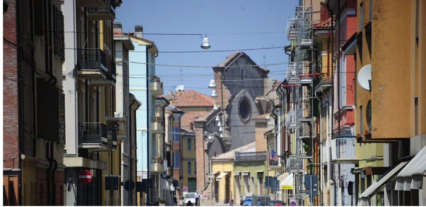
Figure 1: Localized collapse of buildings in Mirandola
