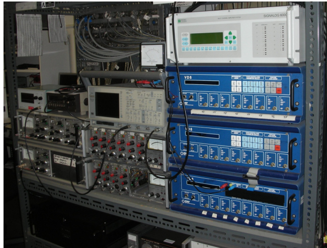
Figure 4.18 External amplifiers for pressure sensors type 1
