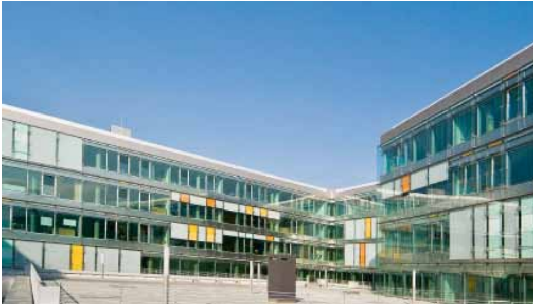
Pic. 32 - Secondary School "Giovanni Pascoli", Bolzano, Project: arch. Ranzani
