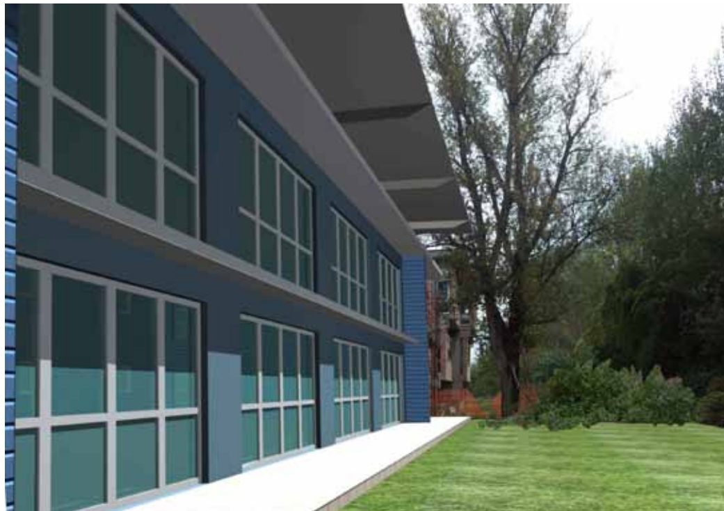
Pic. 03 - South Facade, Majorana Secondary School in Capannari, Lucca. Project: Lucca Administration, 2011
