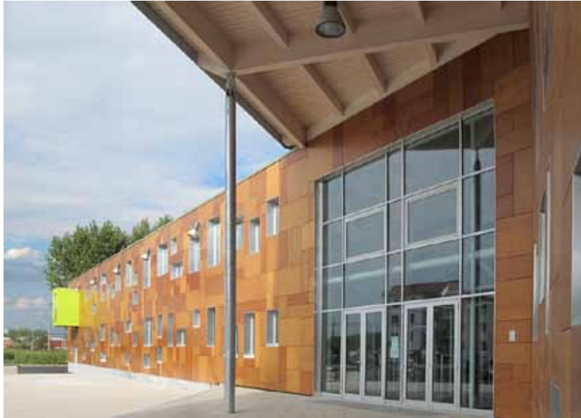
Pic. 60- Piobesi Torinese Elementary School, Archiloco Studio Associato the use of photovoltaic and solar Thermic panels, geothermic and green roof, natural ventilation chimneys low emission glass, permits the school to have a usage of 3,6 kwh/mc/year.
