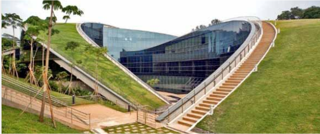
Pic. 23 - The Singapore art school is a building which hosts the Design and Media school and the Nanyang Technological University. The two "hills" with stairs are accessible to students who can enjoy in complete freedom their break moments. Besides establishing an active relation with the surroundings, the natural ceiling functions as insulator and air purifying.
