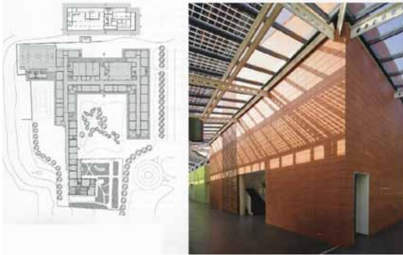
Pic. 10 -The new building uses the brick for both internal and the external environment. The intermediate cover is made of metal and glass with solar integration.
