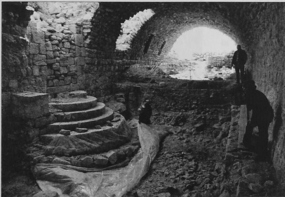
11. Ash-Shawbak. The monumental stairway, discovered in 2006, which connected the vaulted hall of the Crusader palace with the new Ayyubid government palace.
