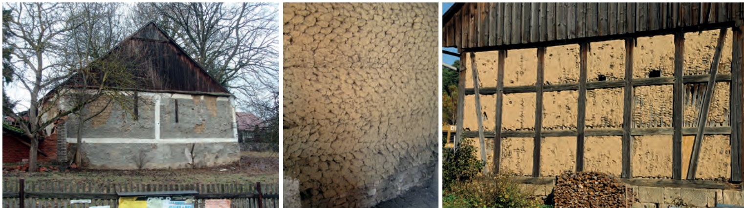
Examples of historical building techniques: adobe masonry, clay rolls opus spicatum, half timbered structures with wattle and clay. (photos: Žabičková Ivana, Růžička Jan)
