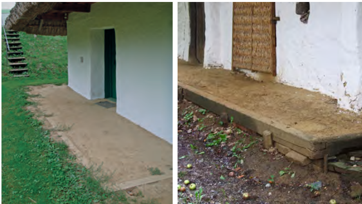
Exterior sidewalk enclosed by timber under thatched eaves in Heiligenbrünn Village. Rammed earth sidewalk enclosed by timber. Traditional house in Heiligenbrünn Village. Reconstruction of the interior space of an earthen house, Gerersdorf Open Air Museum. (photos: Fernando Vegas, Camilla Mileto)
