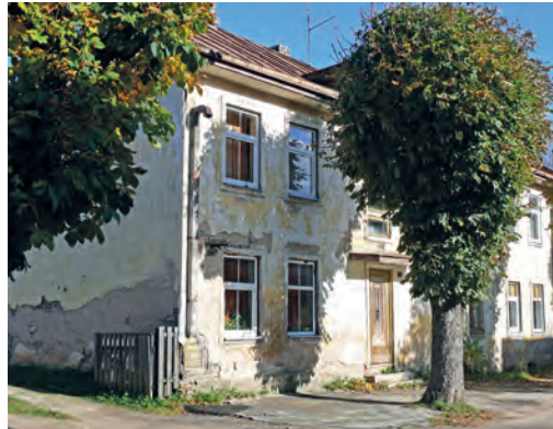
Building in wattle and daub in Tartu, Tartumaa. (photo: René Guérin)
