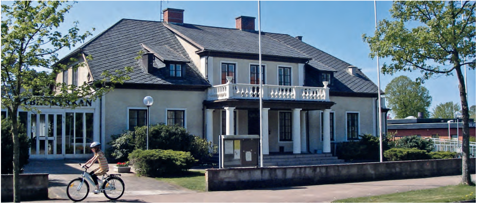
Villa Terra in rammed earth built in 1925. Falkenberg, Sweden. (photo: Jenny Andersson)
