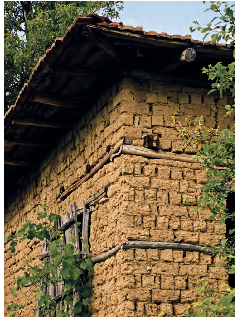
Adobe and wooden timber, house in the region of Gotse Delchev. (photo: Saverio Mecca)
