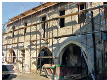
Adobe residence during its restoration
