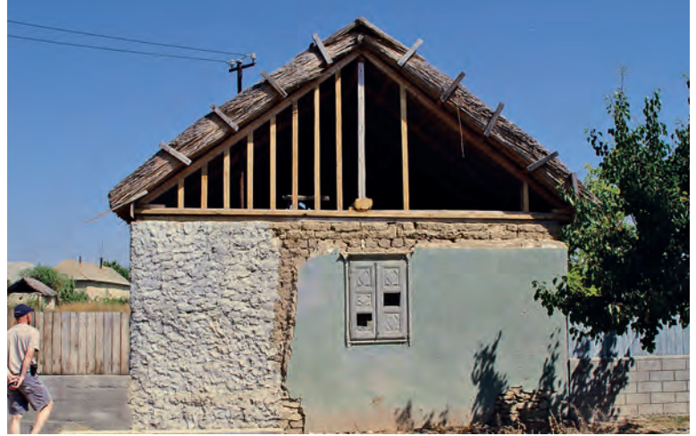
House under renovation in Dobrogea region
