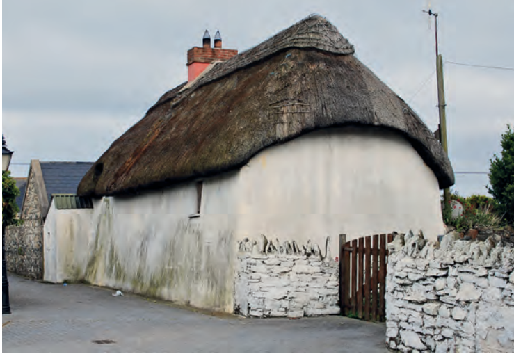
Mud house, plastered with cement / Kilmore Kay, Co. Wexford. The mud house of an old farm / Poulwitch, Mayglass, Co. Wexford. Two storeys mud house, plastered with cement / Next to Kilmore Quay, Co. Wexford. (photos: Marie Chabenat)
