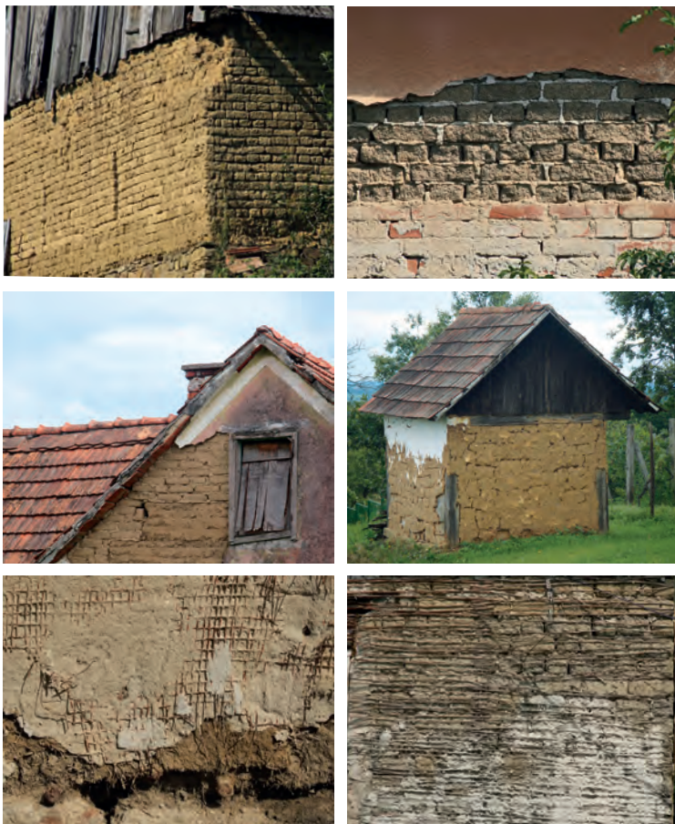
Adobe wall, Czech Republic; Adobe wall, Ziharec village, Slovenia; House detail at Nova vas pri Markovci villaje, Slovenia; Magyarszombata village, Hungary; Wall covering in Ziharec village, Slovenia; Wall covering in Szolnot village, Hungary. (photos: Fernando Vegas, Camilla Mileto)
