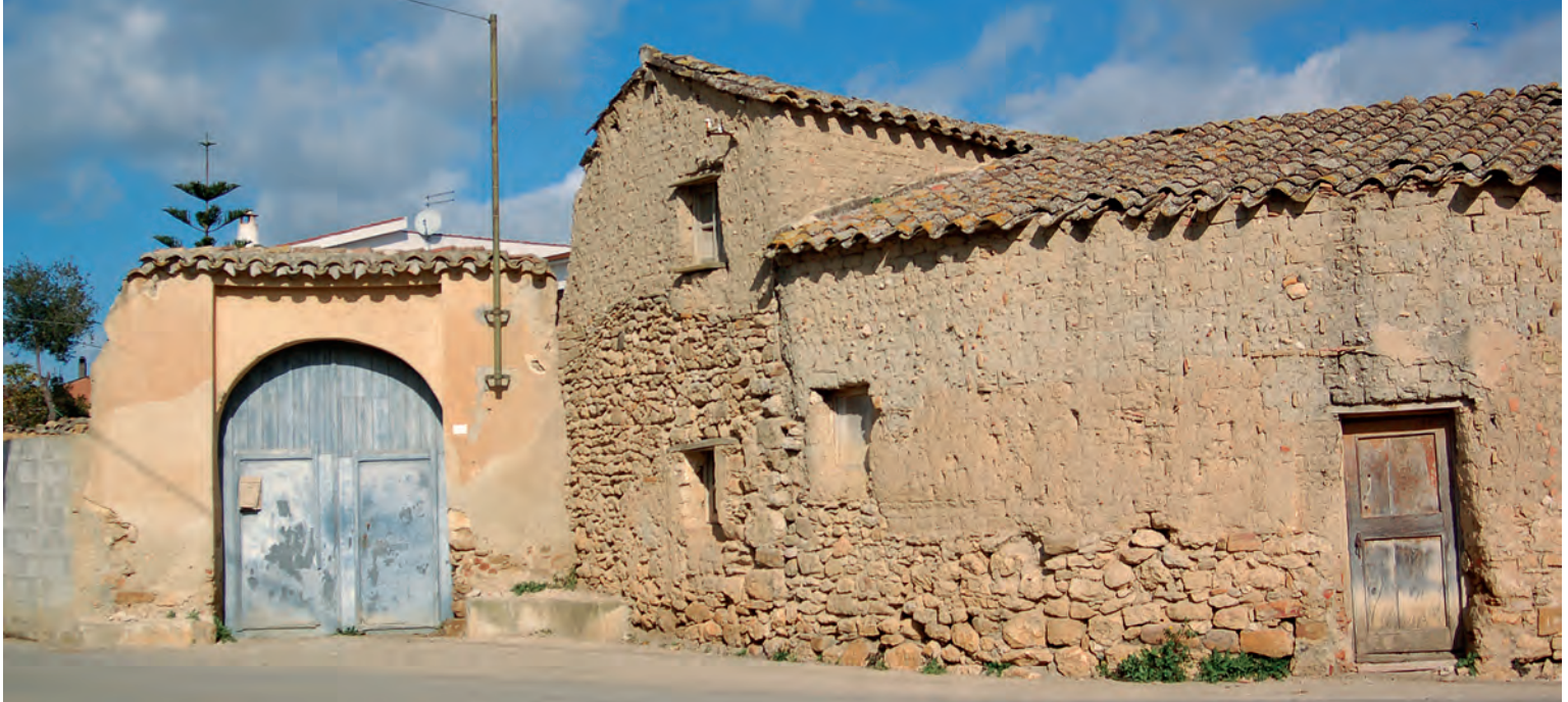
Traditional house in adobe (domu) in Samatzai, Sardinia, Italy. (photo: Silvia Onnis) Adobe houses in Sambiasi, Calabria. (photo: Ettore Pelaia)
