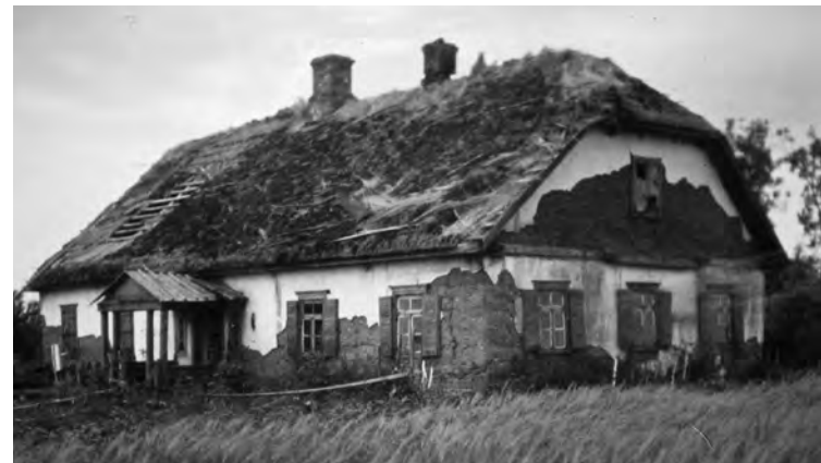
Dwelling house made with wattle clay, Kėdainiai district, second half of XIX century.
