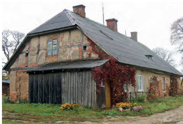
Rammed earth barn in Lielplatone manor, middle of the 19th century, Kurland, Jelgava district, Lielplatone parish. (photo: M. Putniņa)
