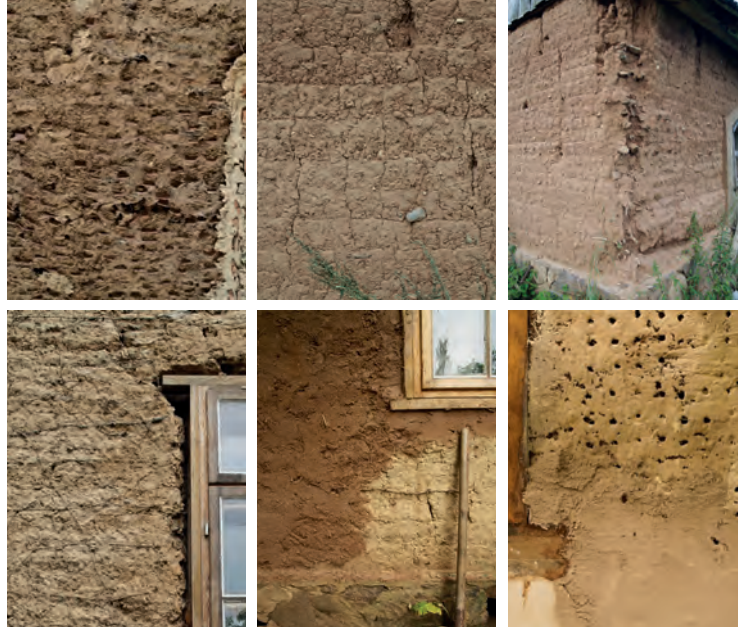
Rammed earth wall construction with fragments of broken ceramic roof tiles. Economy building of Bērzgale manor. Rēzekne district, Bērzgale parish.
