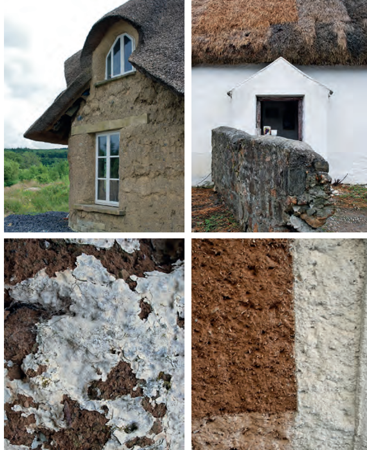
Contemporary mud house (self built) / Owning, Co. Kilkenny. The mud house of an old farm / Poulwitch, Mayglass, Co. Wexford. Farm building/ Limewashes detail / Effin, Kilmallock, Co. Limerick. Sample of lime plasters on clay walls / Traditional Lime Company / Tullow, Co. Carlow. (photos: Marie Chabenat)
