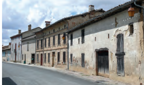
Adobe houses, Salvagnac, Tarn. (photo: René Guérin)
