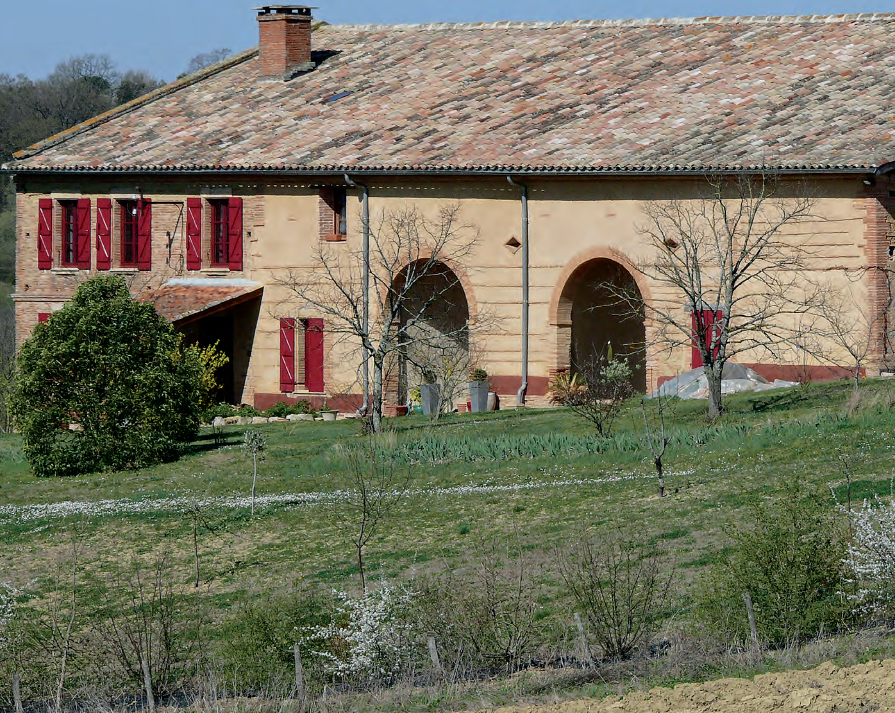
Farmhouse in rammed earth, adobe and bricks in La Salvetat-Belmontet, Tarn-et-Garonne. (photo: René Guérin)
