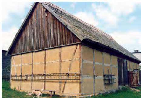
Half timber barn with wattle and daub in fill (XIX c.), Nadole, Pomorze. (photo: Teresa Kelm)
