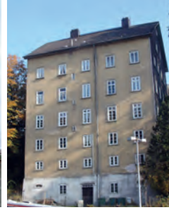
Six-storey building in rammed earth, Weilburg, Hessen. (photo: DVL H. Schreckenbach)
