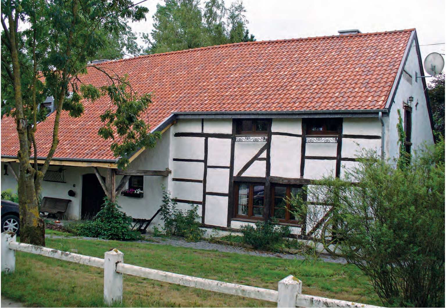
Timber frame and wattle and daub, Belgium. (photo: Jacob Merten)
