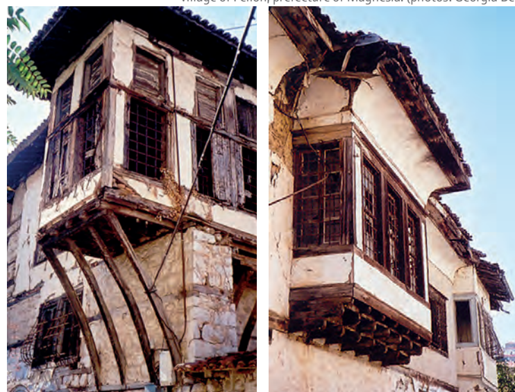
Adobe walls and Sahnissi on the upper floor. Agios Lavredios, village of Pelion, prefecture of Magnesia. (photos: Georgia Bei)
