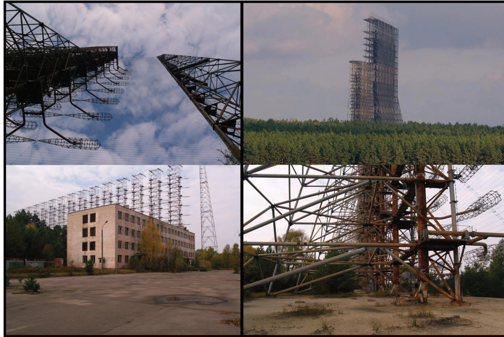
Figure 3.4. Antenna systems of the abandoned soviet OTHR-SW system “Duga-2” that was part of the “Chernobyl-2” radio/radar facility.
