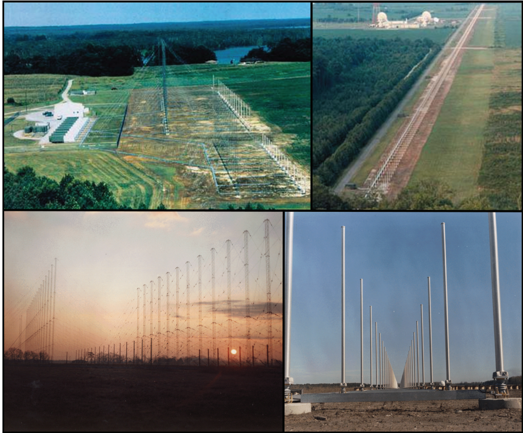
Figure 3.11. Antenna configuration for the transmitting (left) and the receiving (right) arrays of a bistatic US Navy OTHR-SW.
