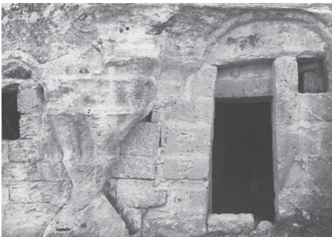
Fig. 11 Main entrance to the church of Saint Girolamo.
