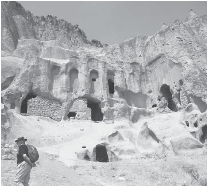
Fig. 23 An example of erosion and wrong human intervention in Selime.
