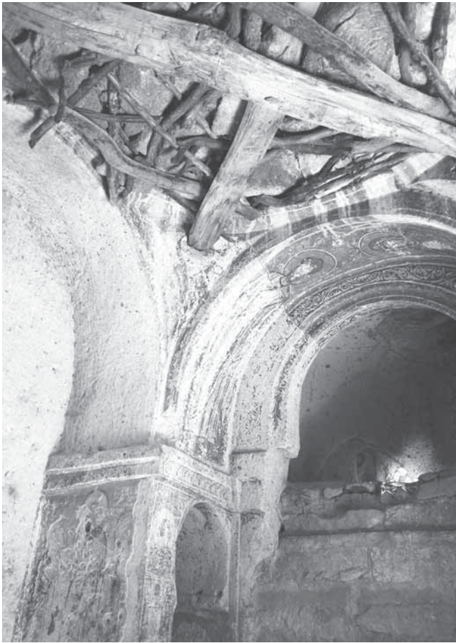
Fig. 15 Nino Kilise. Plugging of the pendentives. (photo: C. Crescenzi)
