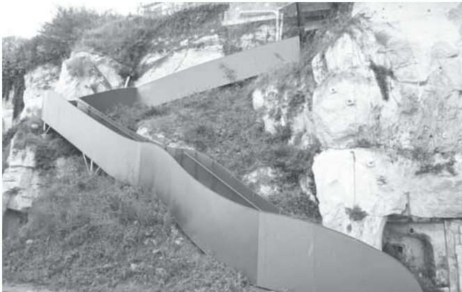
Fig. 12 Outdoor staircase of the hillside.
