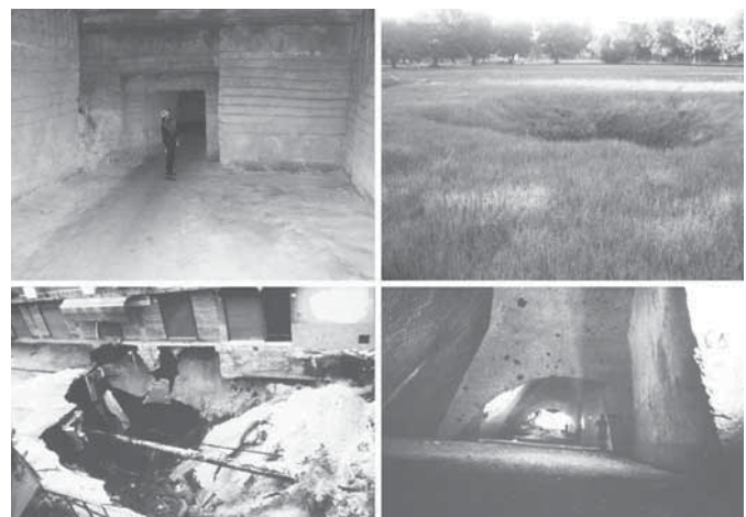
Fig. 18 Examples of underground cavities which have generated sinkhole phenomena (Cutrofiano, top, and Lusignano, bottom) causing, sometimes, serious damage to the overlying rural and urban settings (Cutrofiano photos: M. Parise; Lusignano photos: B. Bocchino, S. Del Prete).
