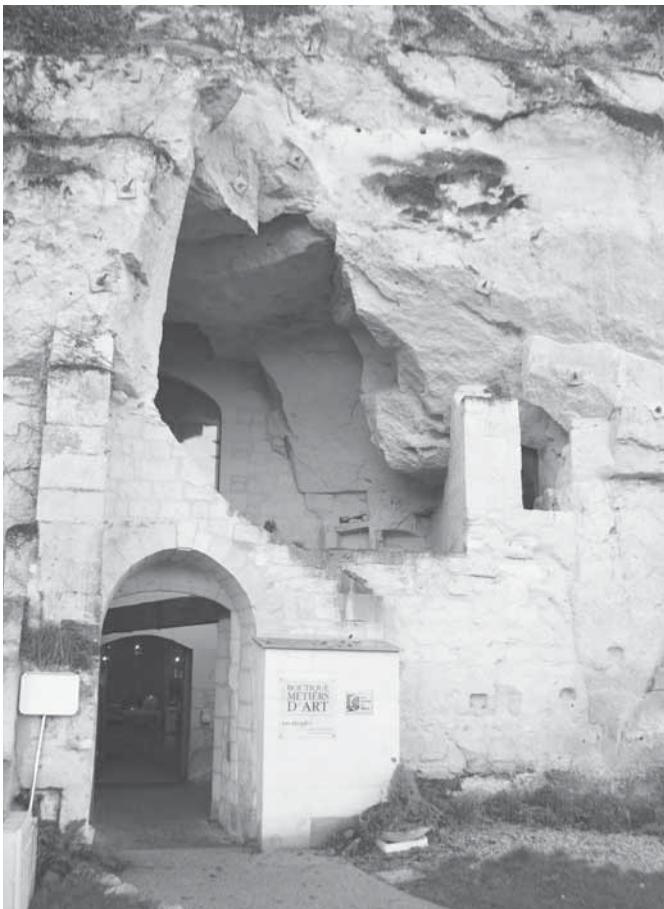
Fig. 13 Façade of the art craft workshop.
