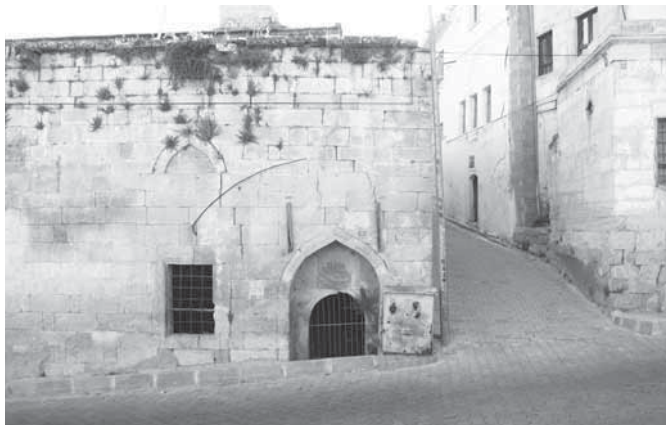
Fig. 22 The street at the north of Alaaddin Mosque, 2011.
