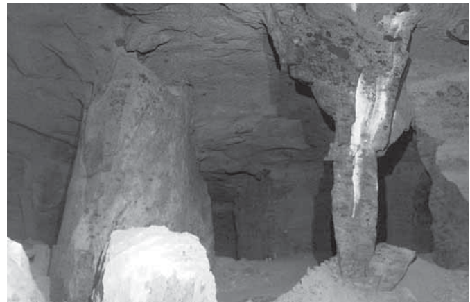
Fig. 17 Internal view of a trachyte mine (Del Prete, 2004) at the foot of Camaldoli hill (Napoli): huge rocks detached from the vault and from the pillars (photo: S. Del Prete). The pillars are evidently compressed by the static solicitations of the loads.
