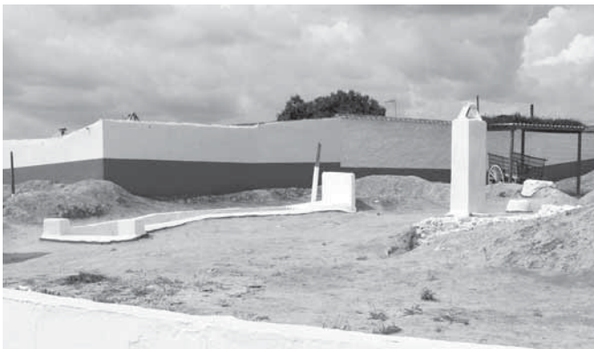
Fig. 3-4 Sunken-feature architecture in Villacañas, Toledo, Spain.
