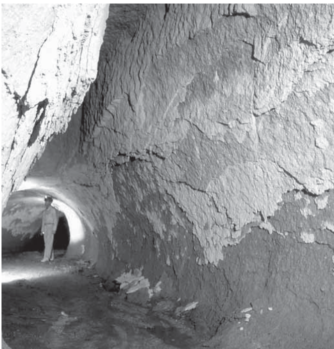
Fig. 9 Meskendir Valley (Cappadocia – Central Turkey). The millenarian erosion in an artificial drainage tunnel has caused the remodelling of the cross section: the original section is suspended on the vault of the cavity (photo: G. Bologna - Centro Studi Sotterranei). In this case, the remodelling is caused also by the exfoliation.
