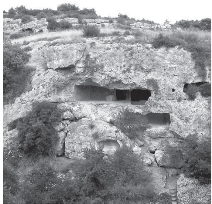
Fig. 16 Madonna della Scala (Massafra, Taranto): the rock failures on the right cliff of the ravine has damaged the caves (photo: M. Parise).
