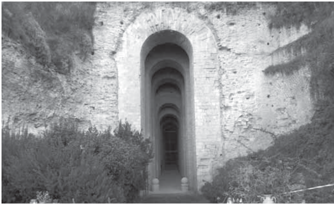
Fig. 2 Entrance of the Seiano Cave between Naples and Pozzuoli. The breadth of the section is less than 2 meters (photo: N. Damiano).
