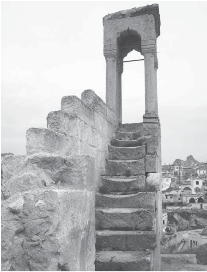
Fig. 15 Çukur Mosque, kiosk type minaret.
