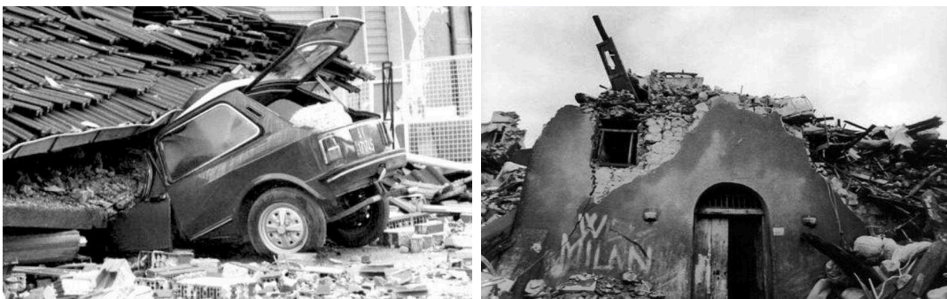
Figure 4: Collapses in the Irpinia territory.
