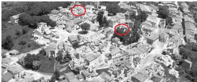
Figure 17: Aerial view of Castelnuovo (AQ) after the 06/04/2009 earthquake. In red, the locations of two collapsed heavy roofs.
