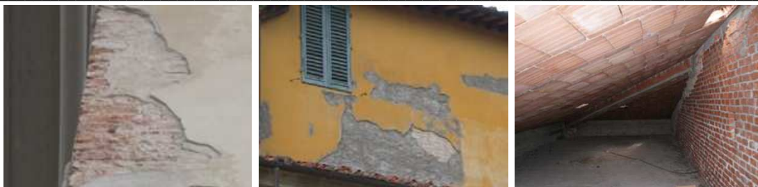
Figure 42: Typologies of masonry and roofs directly observable.
