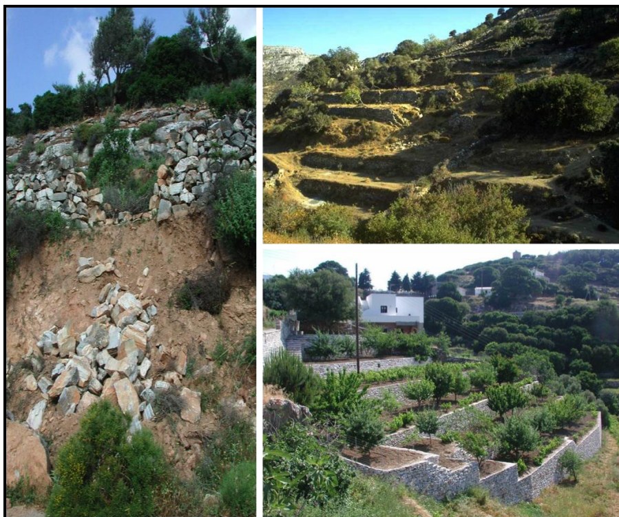
Figure 2: Naxos Terracing Systems in Different State of Conservation. From Left to Right, Clockwise: a Completely Disrupted Terracing; a Poorly Maintained One Which Still Retains Some Protection Efficiency; a Well Maintained System Newly Restored in the Apirathos Area
